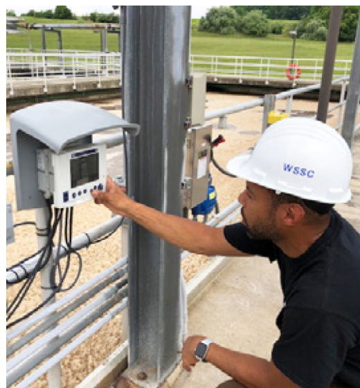
Figure 9: Greg Whitley at the Seneca WRRF using the IQ SENSOR NET system.
