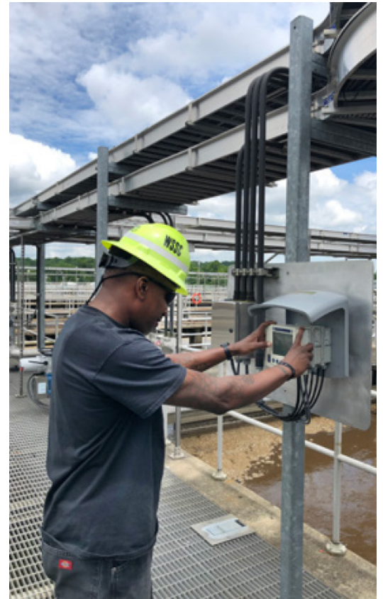
Figure 6: At the Western Branch, Lydell Washington checks real-time nutrient measurements on the IQSN 2020 3G controller.
