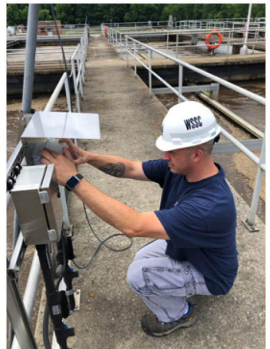
Figure 7: Dave Kramer, Chief Plant Operator for the WSSC Western Branch Facility
